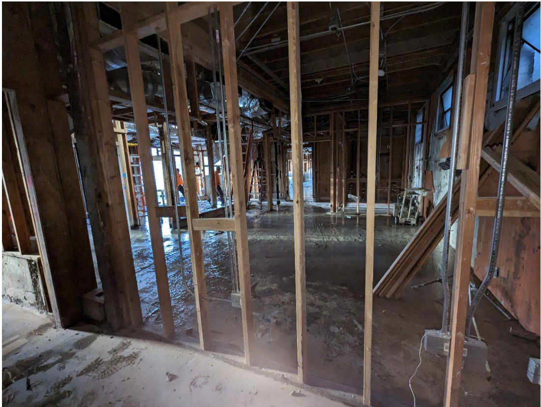
First Floor – Office Areas
