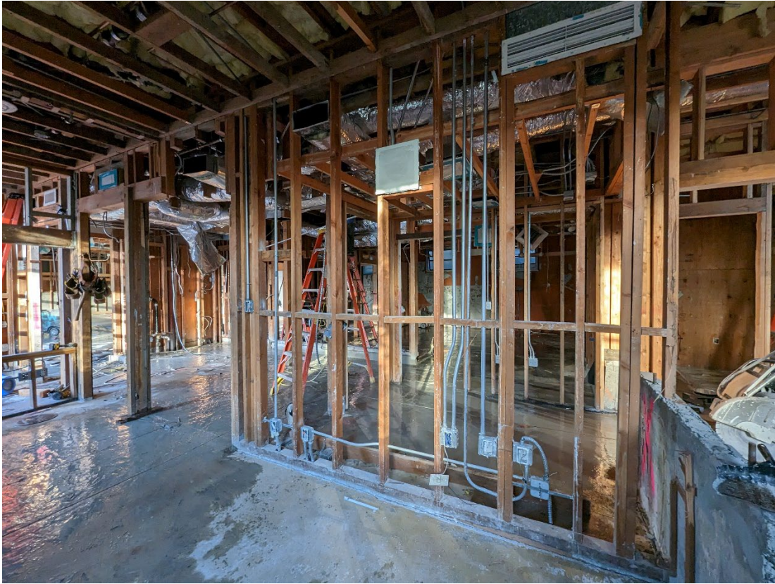
First Floor – Office Areas
