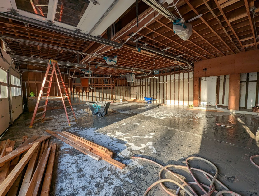
First Floor - Apparatus Bay
