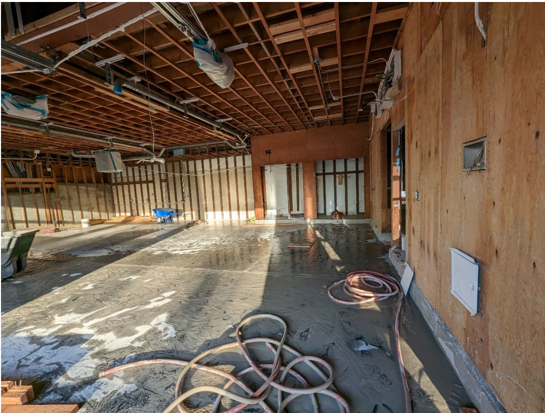
First Floor - Apparatus Bay
