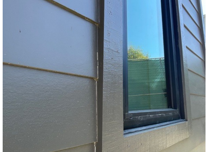
Includes adding/repairing caulking around windows and trim.
