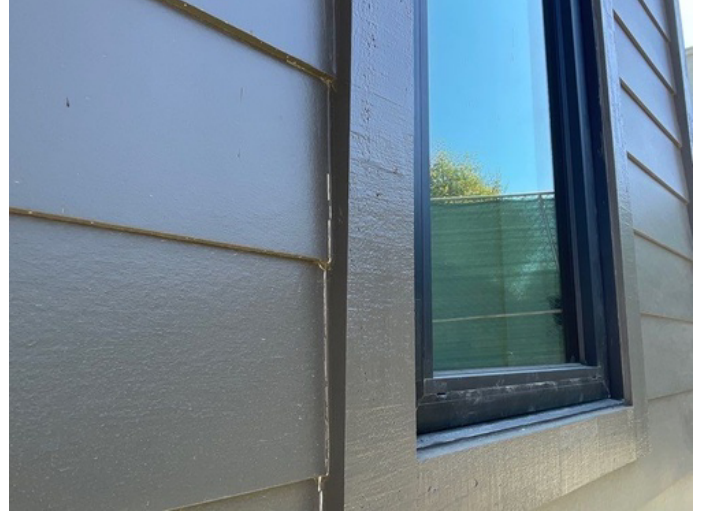
Includes adding/repairing caulking around windows and trim.
