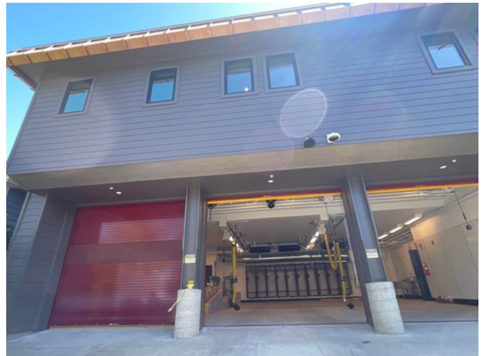
Includes painting eaves, window and door casings, and posts on building. Does not include roll up doors.
