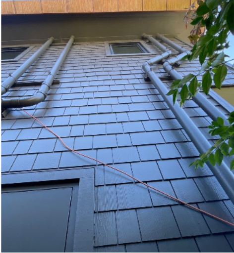
Includes painting the eaves and the conduits.
