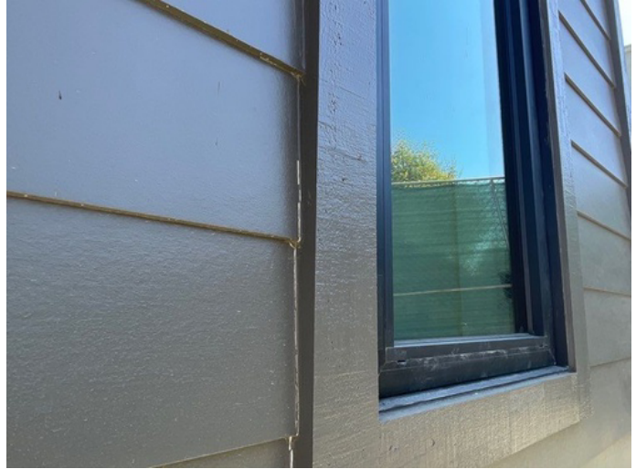
Includes adding/repairing caulking around windows and trim.
