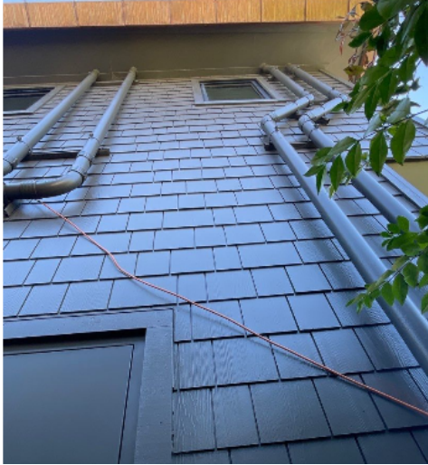
Includes painting the eaves and the conduits.
