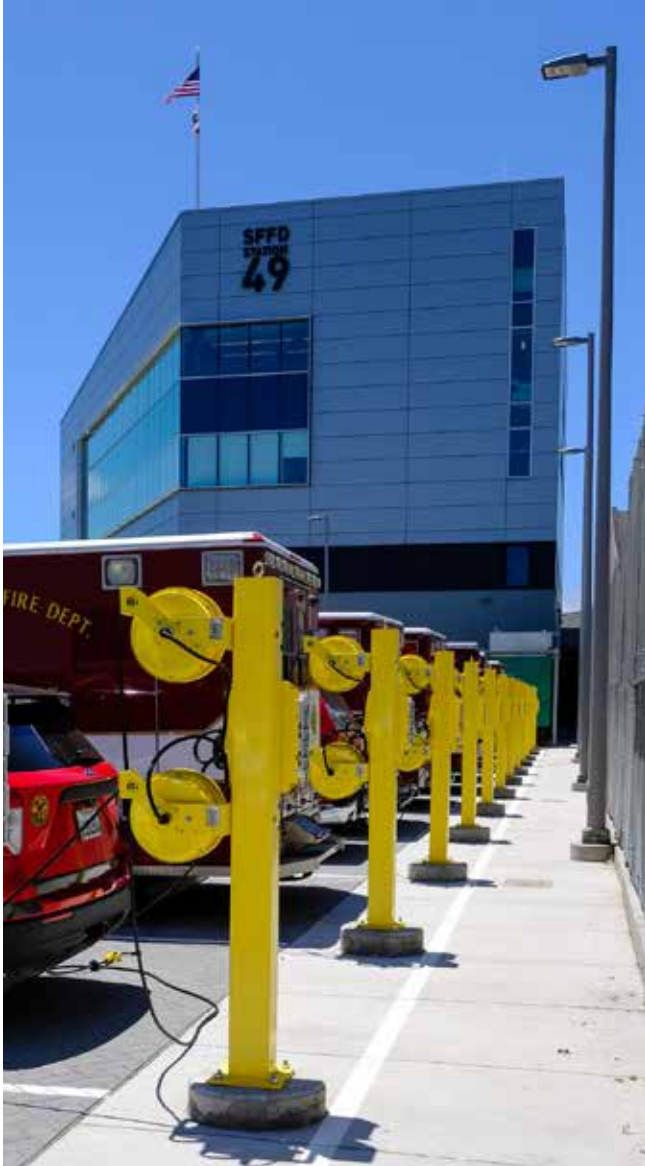
SFFD Ambulance Deployment Facility
