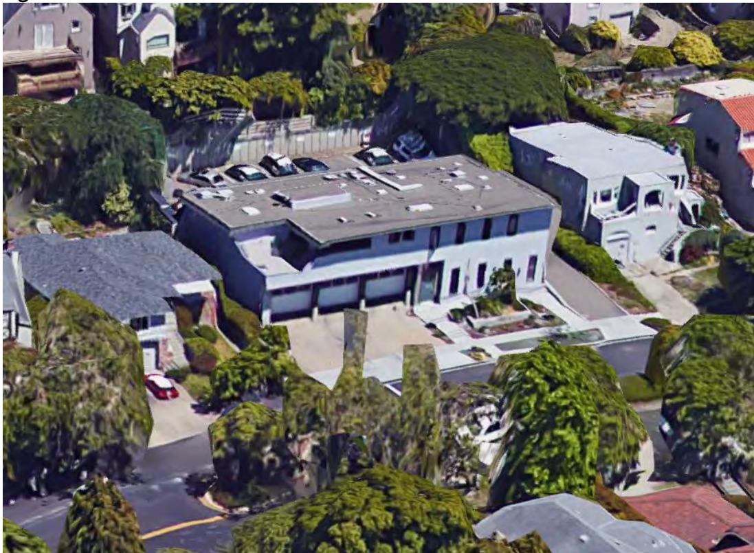
Figure 4: View from the West
