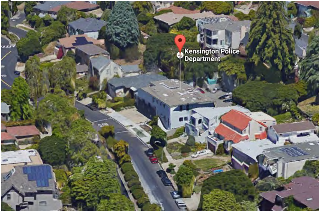
Figure 3: View from the South
